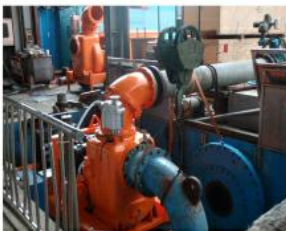
Pump Performance Test
